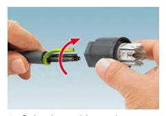
1. Strip the cable and prepare the PE conductor.
